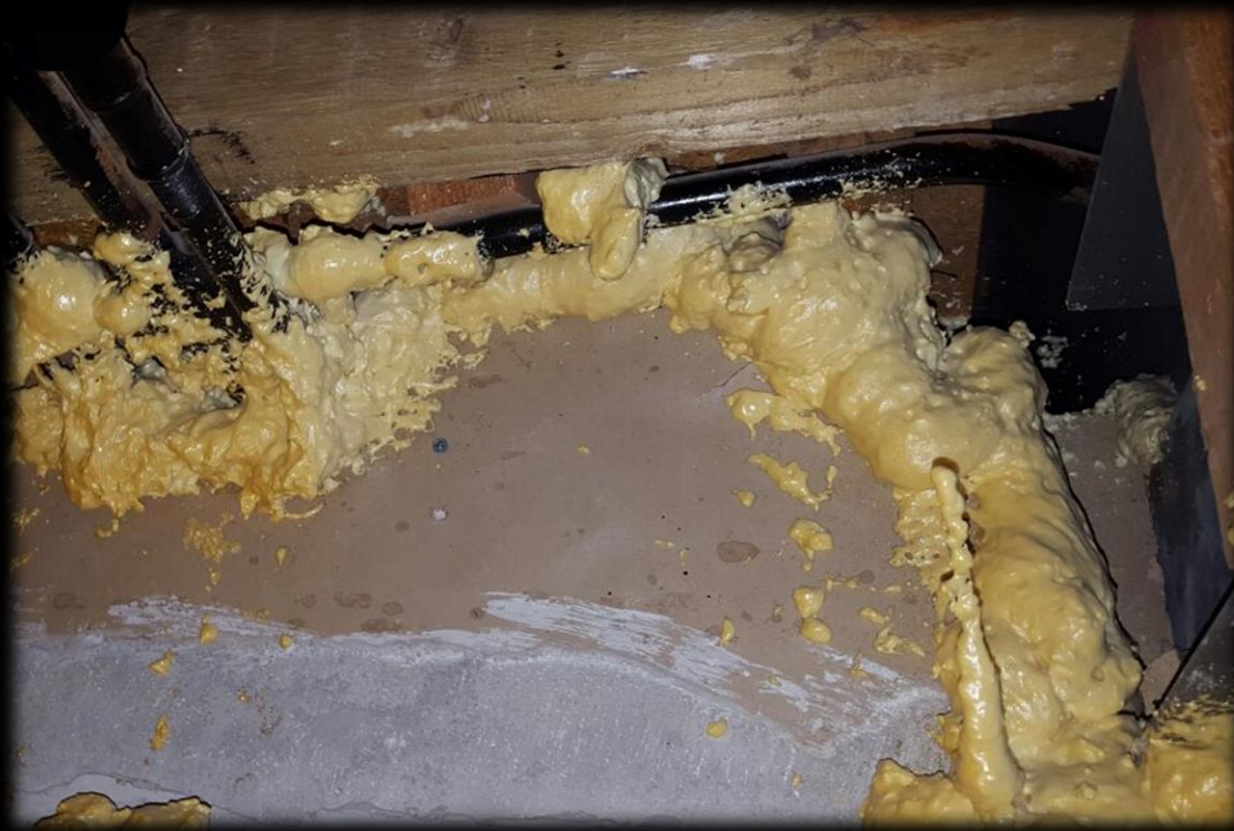
PU foam located in open voids across the property in an attempt to seal larger voids.
